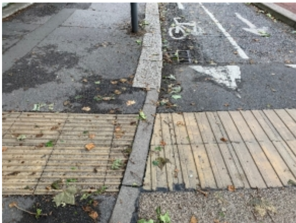
Corduroy used instead of ladder at this shared arrangement transition
