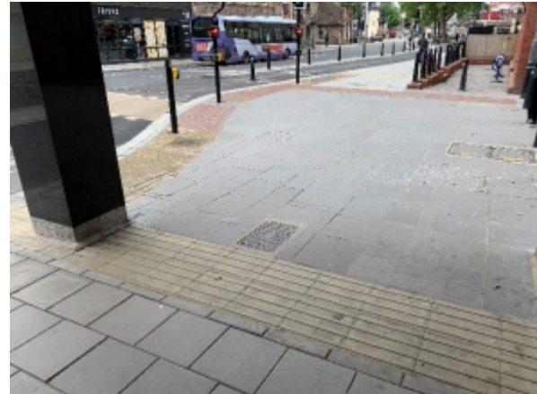
Ladder surface used to denote transition from footway to shared area: should be corduroy
