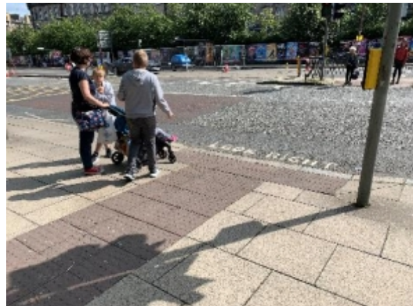
A T-shaped, rather than L-shaped blister paving arrangement at a signalised crossing
