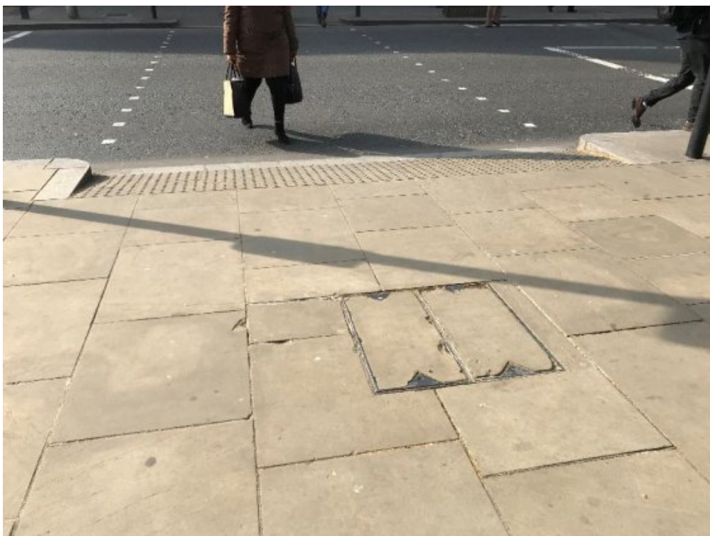
Figure 2: Yorkstone blister/paving at signals in town centre area. No tonal/colour contrast or stem.
