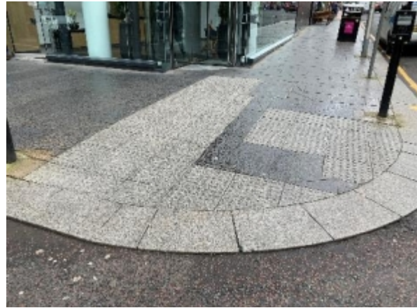
Conflicting blister tails on a flush radius, with the decision taken to cut one very short
