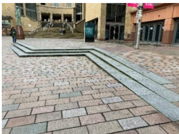
'Fading' steps with no corduroy or other tactile indicators
