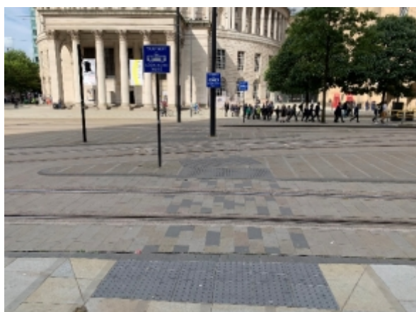
Linked crossings of tram tracks; interstitial footway pattern attempts to give additional visual clues
