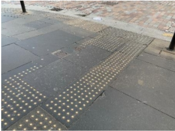
Metal stud blisters used for a stem but with two stud-free slabs inset to the arrangement
