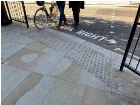
Poorly contrasting curved arrangement: uniform 800mm depth avoids wedges; but no stem
