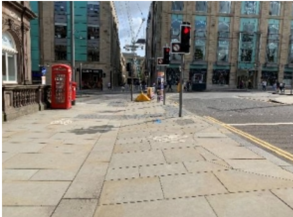
Start of a shared walking/cycling area with no tactile indicators
