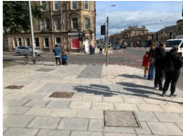
Non-contrasting blisters at perpendicular crossings, with both stems ending in open space
