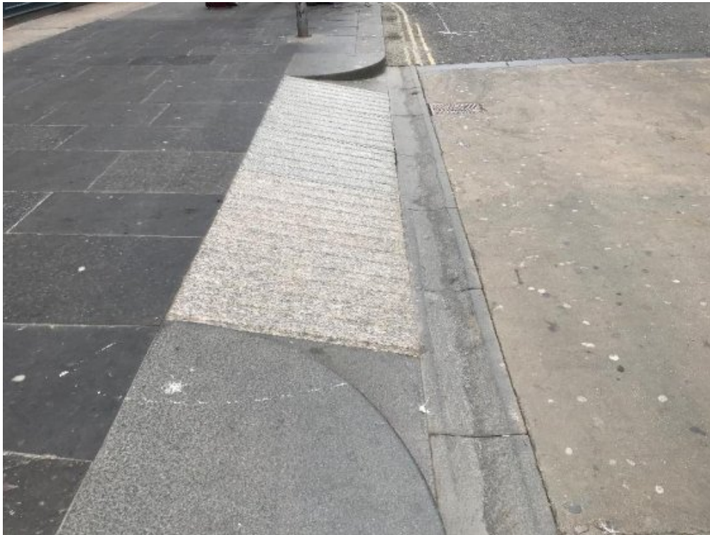
Figure 3: Non-standard quasi-tactile paving at signals in heritage area. No stem. Some tonal contrast. Steep gradient.
