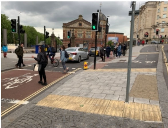
Non-compliant use of tramline and ladder at closely-associated controlled and uncontrolled crossings.
