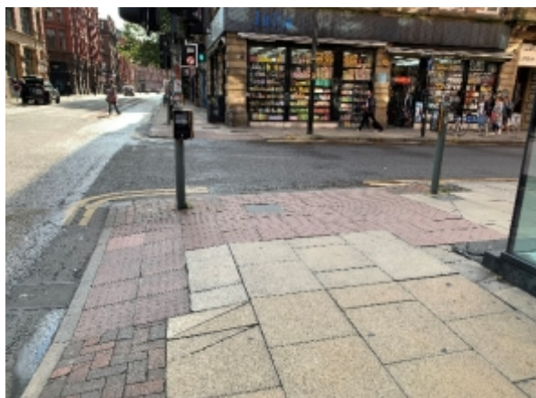
Confusion between stems at closely-associated perpendicular crossings.
