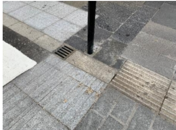
Corduroy as cycle path edge marker, next to ladder used as rumble strip, and blisters at cycle path zebra
