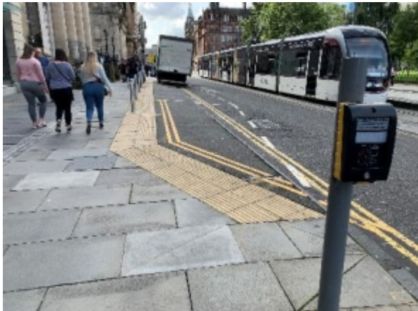
Corduroy paving (800mm depth) used to warn of a loading bay at footway level
