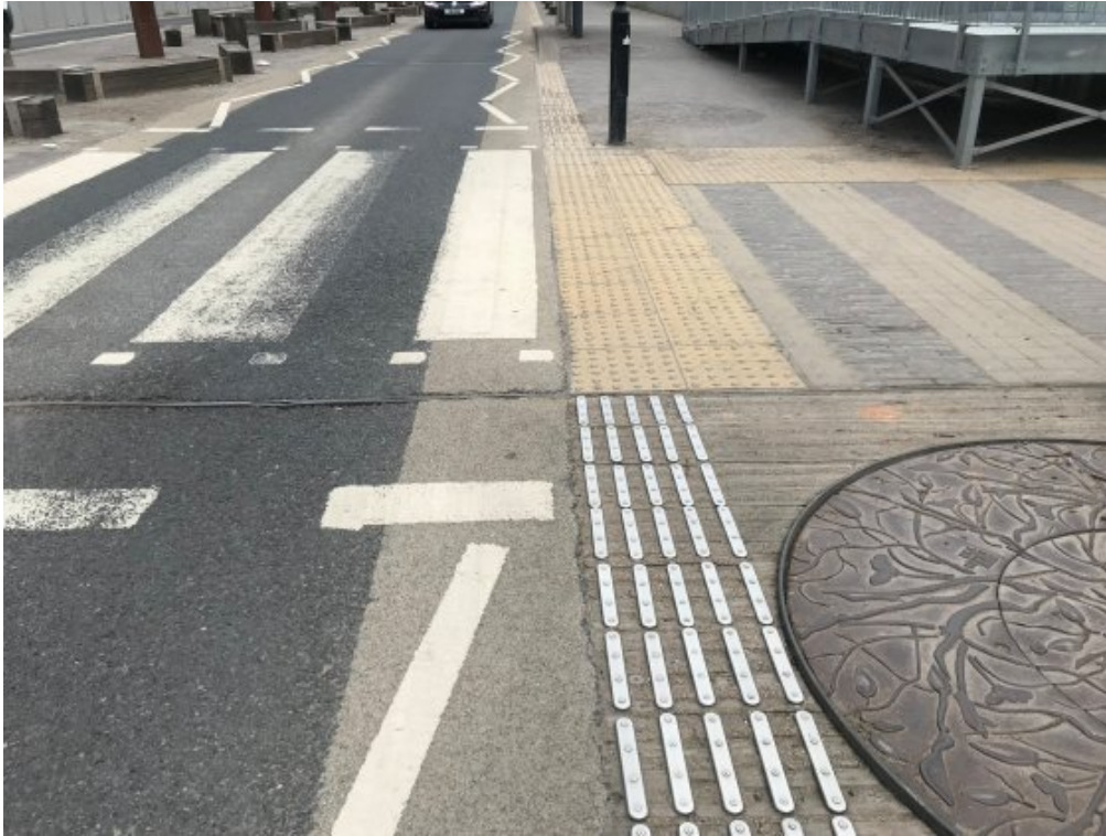
Figure 7: Guidance path surface used as a carriageway edge marker; buff, not red, blister paving used at a zebra.
